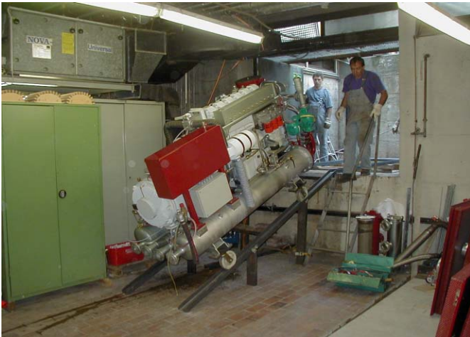
Installation of the CHP
