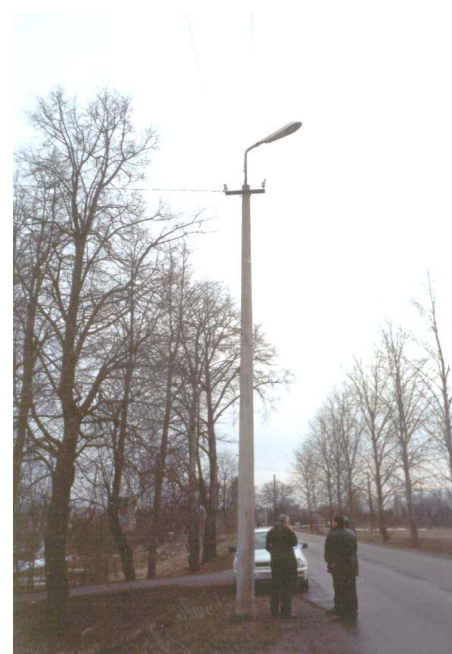
Figure 1: Concrete pole in Raudas street - Tukums
