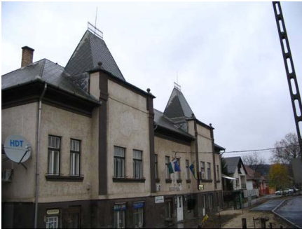
Mende (Pest County, Hungary), Building of Municipal Offices
