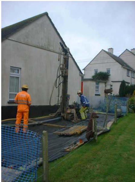
Drilling a borehole
