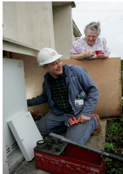
Engineer working on heat pump in external enclosure
