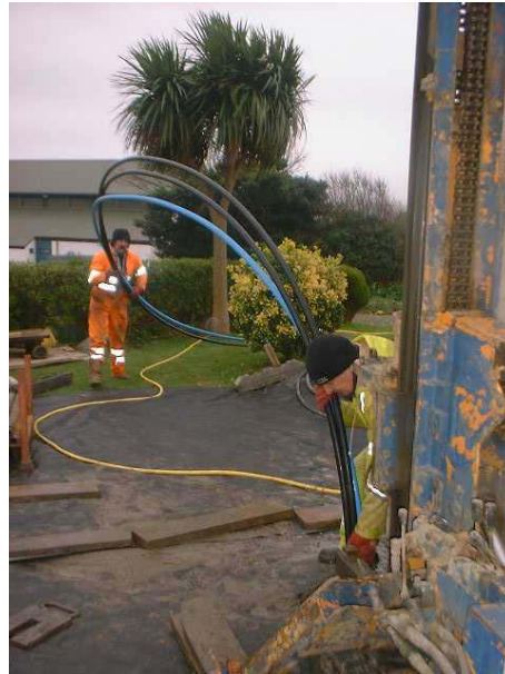
Installing ground loop
