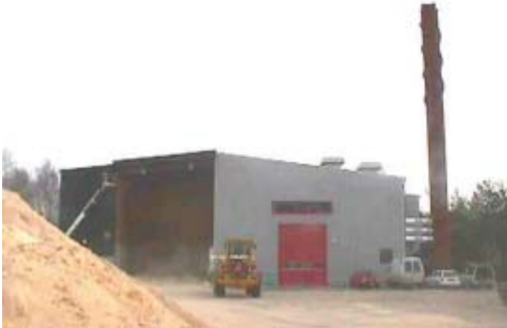
Fig 2 9 MW plant in Braås, one of the largest plants in the project Nearby heating Kronoberg.
