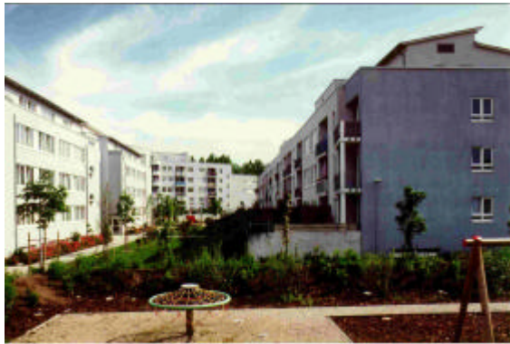
Figure V-I: One of the first improved energy-housing projects in Frankfurt (Specific heat demand: 300 MJ/m 2 a)
