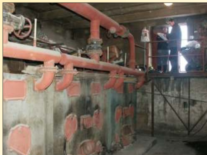
Boiler room before reconstruction
