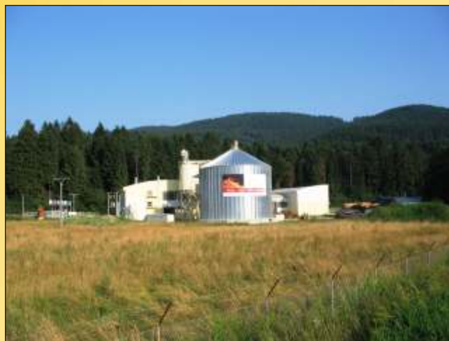
Pellets production plant in Kysucky Lieskovec
