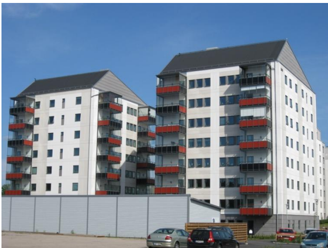
Passive houses in Växjö
